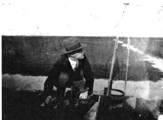
Figure 4-31 (left): Connecting the fuse (electrical ignition cable connected with the auto-support).*
