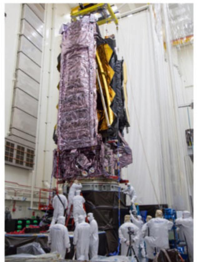
LEFT: The JWST is lifted in folded configuration onto a stand in the clean room at Goddard Space Flight Center April 20, 2017. The primary mirror's "wings" are tucked back and the secondary mirror is also stowed, mounted to the two support struts straddling the center of the primary. NASA/CHRIS GUNN
