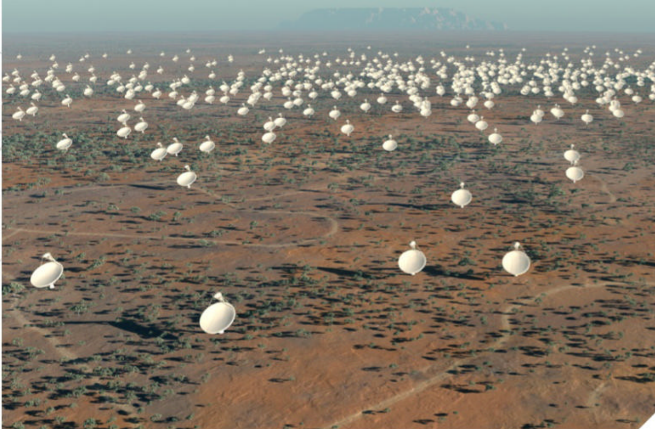
The Square Kilometre Array is envisioned to eventually consist of some 2,000 radio dishes across Africa (pictured here as a photoillustration) and up to 1 million antennas in Australia. Even in its smaller initial form (which is currently under construction) of roughly one-tenth that size, it will generate up to 1 terabyte of data per second. SPDO/TDP/DRAO/SWINBURNE ASTRONOMY PRODUCTIONS/CC BY 3.0
