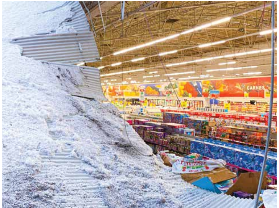
The collapse of the reinforced-sheet-metal roof of the Mega supermarket was the most serious damage caused by the hailstorm in Mexico City on 12 June. No injuries were reported. Credit: Hector Dorantes
