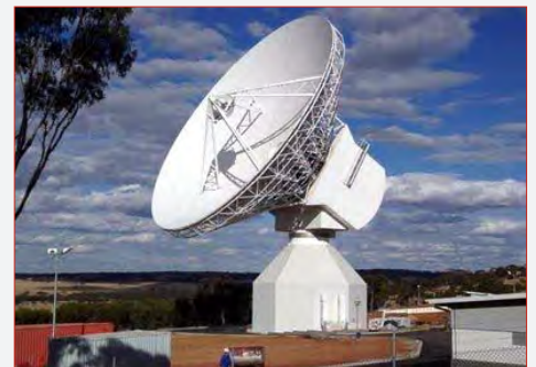
The New Norcia station DSA 1 (Deep Space Antenna 1) is situated in 140 km distance north of Perth. The site hosts a 35-metre deep-space antenna with transmission and reception in both S- and X-Band. (Credit: ESA)
