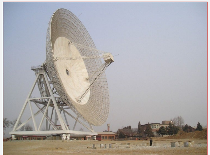
The newly built 64 m antenna in the Jiamusi deep-space tracking station. (credit: Chinese internet)
