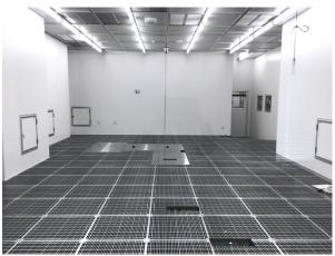
Fig. 2. A newly renovated clean room for O-REx returned samples. Its cleanliness level is ISO 6. It has a grating floor and a base for new CCs, which is under development and will be installed there in fall 2023.
