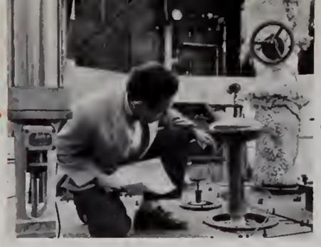
Flow testing of Liquid Nitrogen pressurizing system
