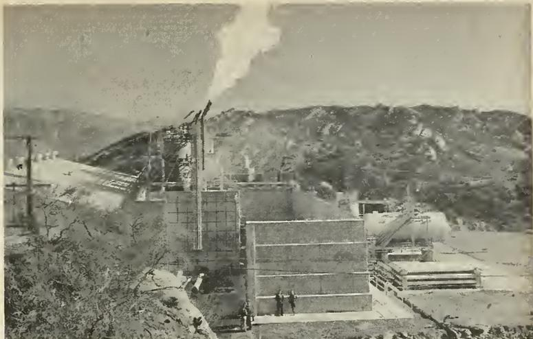
THOR's 135,000-pound thrust power plant is made by Rocketdyne Division of North American Aviation, Inc. Here, rocket engine gas generator flares at Rocketdyne test facility.
