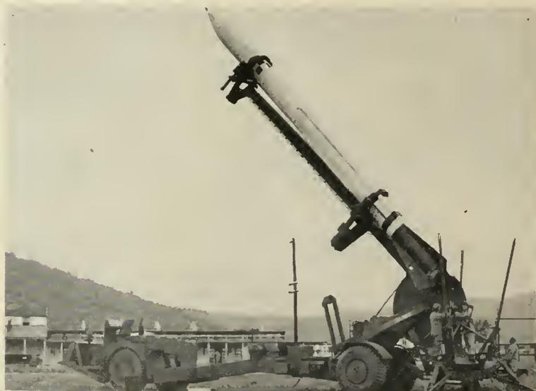
LEFT—CORPORAL leaves launcher in a burst of flame from burning acid and aniline. The missile has a range of about 100 miles. ABOVE—Missile is erected on launcher.
