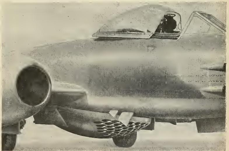
Swiss Oerlikon's bid in the small air-to-air folding fin rocket field. This launcher for 76 of the five centimeter diameter projectiles is mounted on a British Gloster Meteor twin jet fighter. Some pilots prefer the straight ahead firing of this center mount to the converging pattern obtained when the rockets are fired from wing-tip pods.
