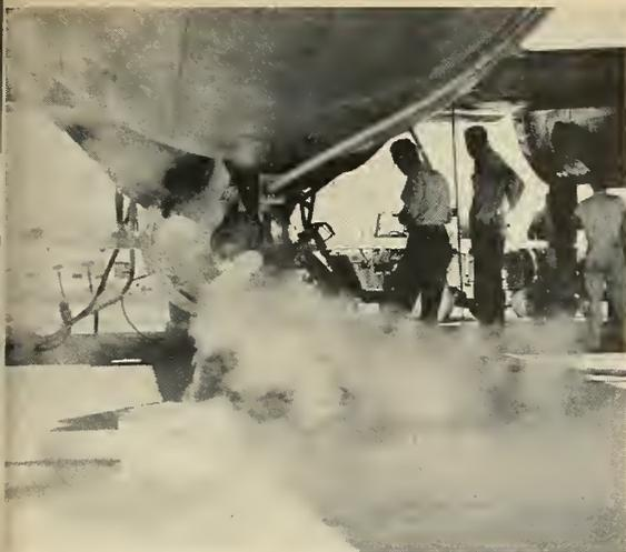
Oxygen is vented to the atmosphere as propellant tanks are being topped prior to takeoff. X-IE has fuel supply for about four minutes. The aircraft obtained a maximum velocity of Mach 2 plus during the first flight. No speed record run was attempted.
