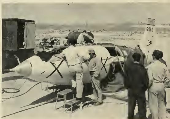
Airplane is readied by NACA, Bell and RMI engineers. First flight lasted for a few minutes and was successful. Landing gear was slightly damaged at landing, delaying the second flight.
