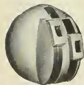
Magnesium turret enclosure for a bomber. Design, lofting, prototypes, production fabrication and assembly are all done by B&P.
