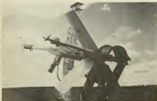
Aft view of the DART positioned on field launcher ready for firing.
