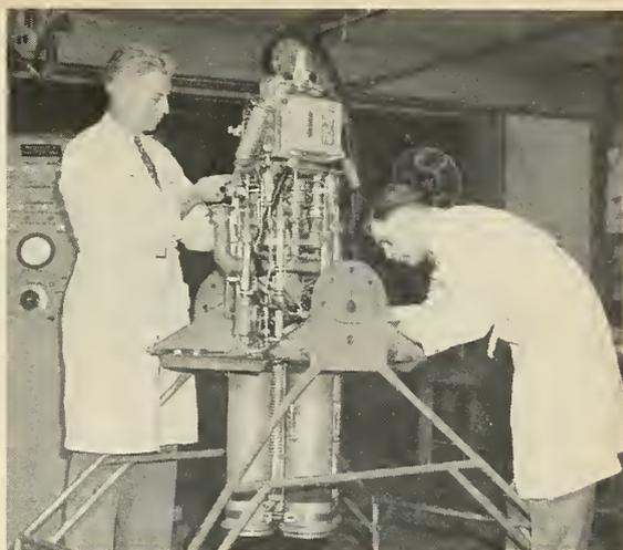
RMI employees, John Wickstead, left, and Holbrook Smith, perform operational check on the 6,000 lb. thrust engine in preparation for test firing. Engine used in the X-IE is designated XLR11-RM-11, basically the same as the one used in the original Bell X-1.
