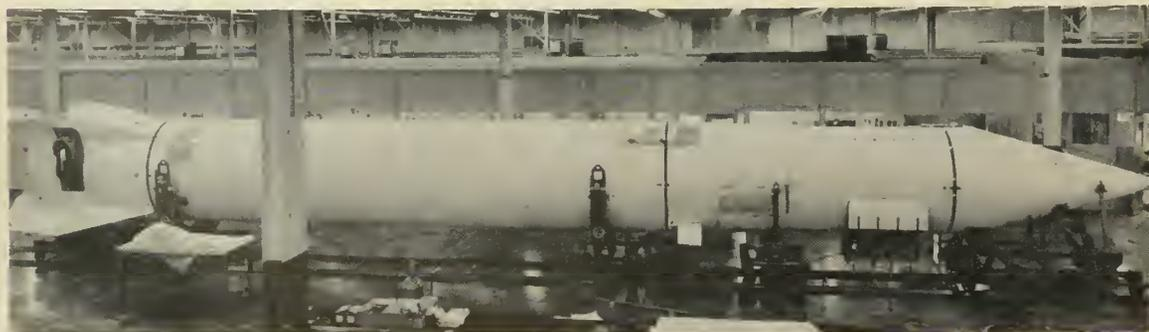
Monitor of aggression . . . giant rocket, Army's REDSTONE, 300-mile missile has just rolled off the assembly line of Chrysler Corporation's Missile Operations. Note the dollies on fixed rail lines, two for warhead and two for engine indicating assembly sequence.
