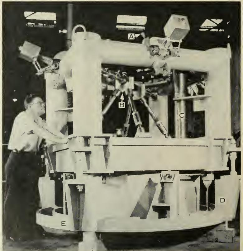
VANGUARD launching and static test platform, manufactured by Loewy-Hydropress, as it awaited shipment to Patrick AFB, where it has been installed for some weeks. (A) Pull-away pickup points on which the rocket rests, (B) the tripod which supports the engine, (C) pipe to carry exhaust to flame deflector, (D) one of four load cells to weigh rocket, fuel, measure thrust and similar functions, and (E) weighing ring for the entire unit.
