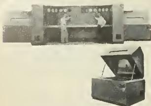
ENVIRONMENTAL CONTROL PANEL AND TWO COLD BOXES USED TO ATTAIN TEMPERATURES FROM AMBIENT TO  $-65^{\circ}\text{F}$  IN MISSILE CONTROL COMPONENTS.
