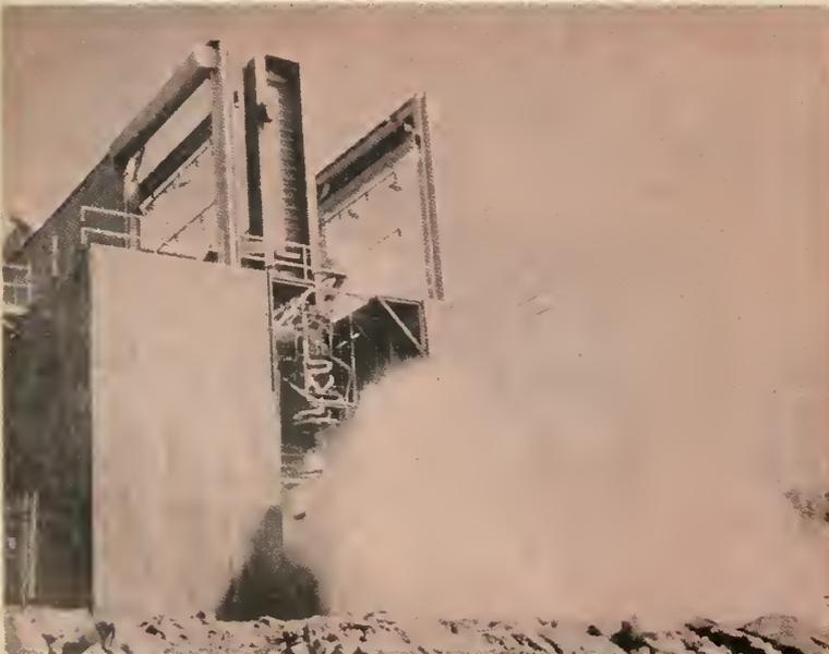
One of the world's more highly developed liquid rocket engines—Reaction Motor's power plant for the North American Aviation X-15 rocket research plane undergoing static test.
