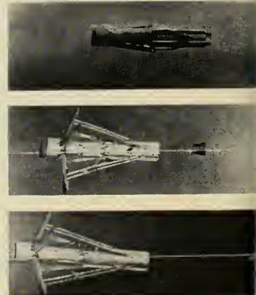
Free-flight tests of missile nose cone models are conducted by GE through use of the separation device. Fired from a five-inch gun, the device extends flaps into the stream, allowing the nose cone model to continue in free flight. This same principle may be applied to large-scale free flight.
