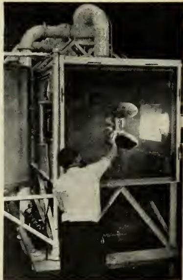
A FIREFLASH is examined after it has been exposed to a simulated dust-and-sand storm for an hour.
