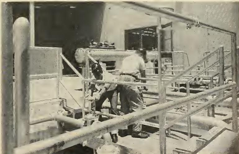
Mechanics Walter Pressir and J. W. Stewart set water-flow control valves on Rocketdyne's high flow bench used to test fuel control components in large liquid fuel rocket engines.
