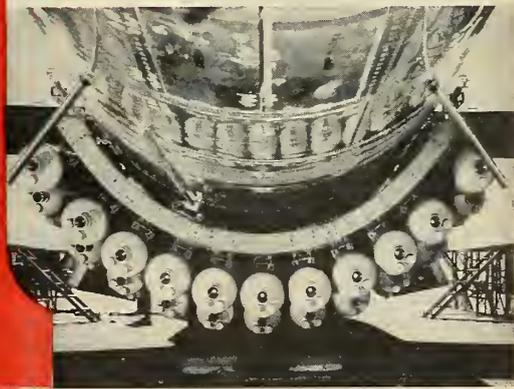
The M15 JATO loaded on Boeing B-47. The first JATO to meet rigid Air Force performance tests. (Boeing Airplane Company photo.)
