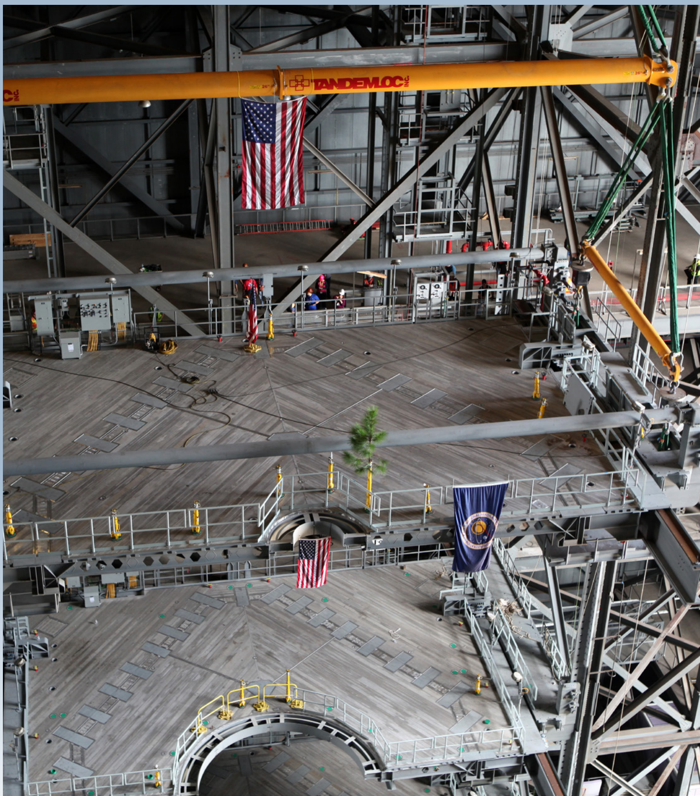
High up in the Vehicle Assembly Building (VAB) at Kennedy Space Center, a crane lowers the final work platform, A north, for installation in High Bay 3. The platform was installed and secured on its rail beam high up on the north wall of the high bay. In view on the platform are the American flag and a small tree. The installation of the final topmost level completes the 10 levels of work platforms, 20 platform halves altogether, that will surround NASA's Space Launch System rocket and the Orion spacecraft and allow access during processing for missions, including the first uncrewed flight test of Orion atop the SLS rocket in 2018. Photo credit: NASA/Frank Michaux
