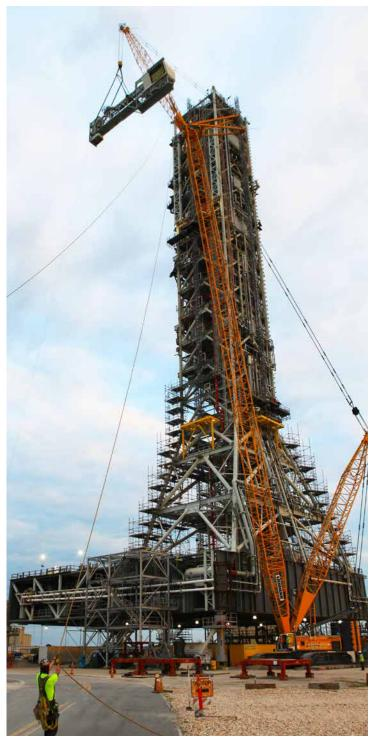
A crane positions the Orion crew access arm so it can be attached to the mobile launche (ML). The arm will be installed at about the 274-foot level on the 380-foot-tall ML tower. Photo credit: NASA/Bill White
