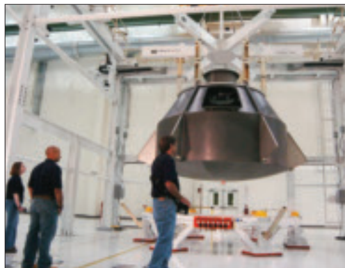
A production assembly crew lowers a full-scale Orion mockup onto the crew module holding structure during an assembly pathfinding maneuver at the Operations & Checkout Facility at NASA Kennedy.
