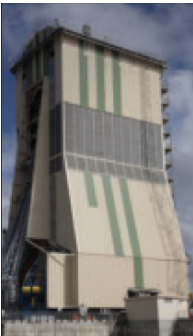
Construction is ongoing for the Soyuz launches in French Guiana. Photographer: Aleksey Yakunin.
