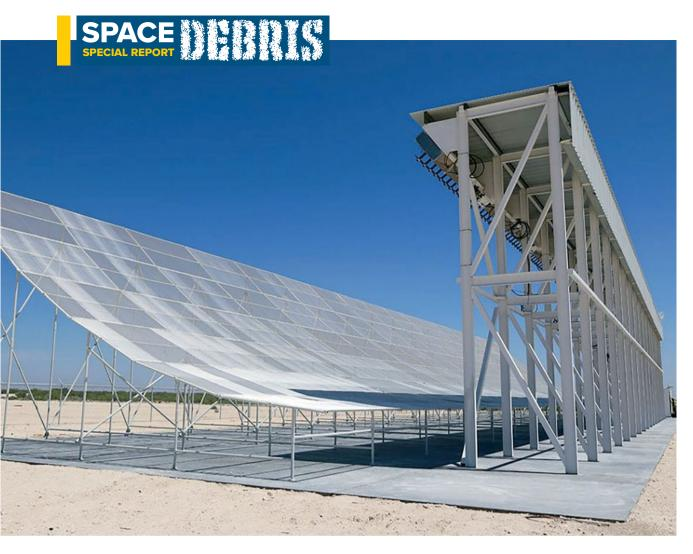
▲ LeoLabs currently operates four radars, including this one in Midland, Texas. The company plans to eventually operate 20 to track pieces of debris as small as 2 centimeters.
