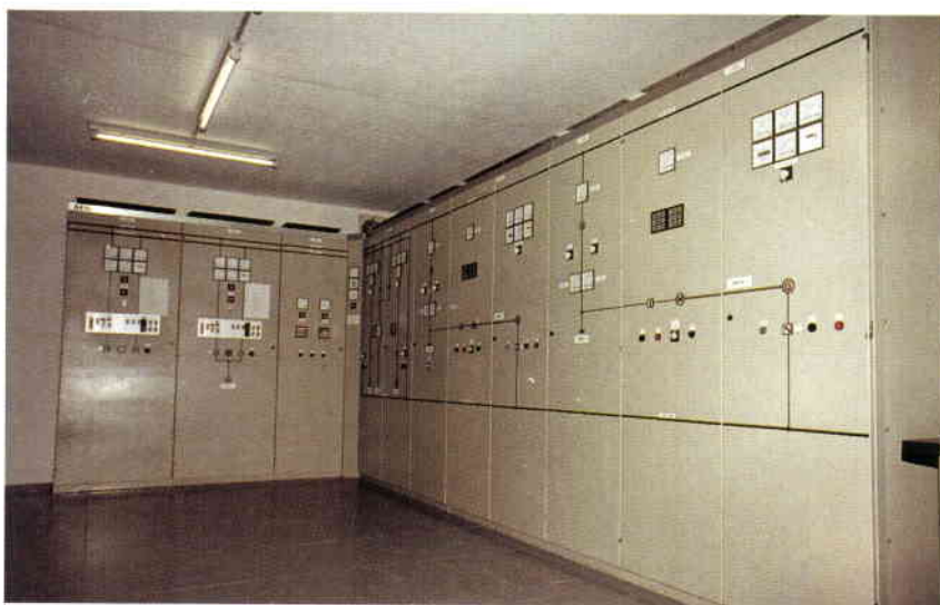
Figure 7. Power-plant control panel
