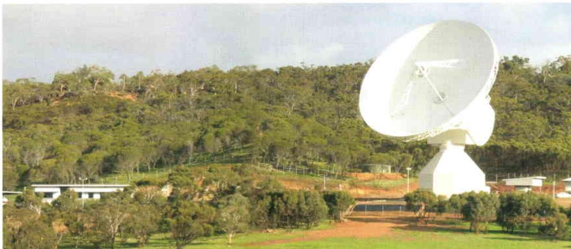
*The New Norcia ground station in Western Australia. Rosetta operations will be controlled from ESA's European Space Operations Centre (ESOC) in Darmstadt, Germany. Signals from the Orbiter will be relayed to ESOC via the 35 metre antenna at New Norcia and a similar one that is currently under construction at Cerebros in Spain*
