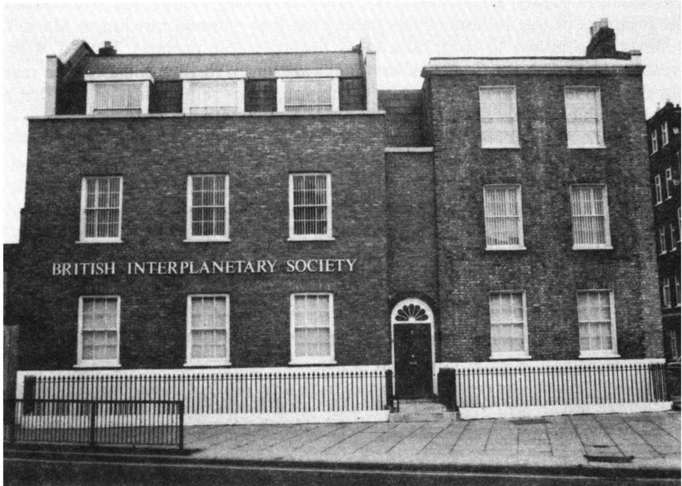
Figure 2 Present BIS Headquarters (1979) at 27/29 South Lambeth Road, Vauxhall, London, SW8 1SZ.
