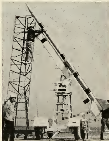
PHOTOGRAPHS AND DATA on the latest Japanese sounding rockets indicate a remarkable advancement in the state of the art. Both of the rockets shown were developed by Professor Hideo Itokawa, Institute of Industrial Science, University of Tokyo. Itokawa is head of Japanese IGY sounding rocket program. K-150 rocket (left). Single-stage, solid propellant sounding vehicle fired April 8, 1958. Diameter—150mm. (5 \frac{1}{2} in.); length—3.3m (10 \frac{3}{4} ft); weight—70kg (154 lbs). Kappa Type V two-stage rocket (right) fired April 29, 1958. First stage diameter—220mm (8 \frac{5}{8} in.). Second stage—K-150 rocket. Maximum velocity—about 1,000 m/sec (3300 ft/sec).
