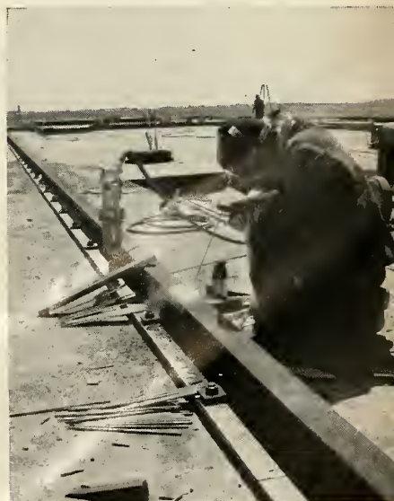
WELDER IS APPLYING finishing touches to the rails that will guide the huge servicing gantry handling the Atlas .
