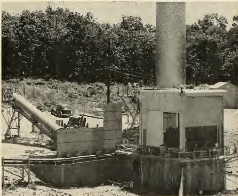
READY TO BEGIN static testing of the Pioneer rocket engine for the X-15 research aircraft is this new concrete and steel test stand built by Reaction Motors division of Thiokol Chemical Corp. The sloping tank (at left) is one of two propellant tanks which are an integral part of the stand. The large tank (background) is the division's 150,000 gallon water tank which supplies the entire test area.
