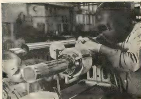
MODULAR connections and bellows permit expansion and contraction of lines.
