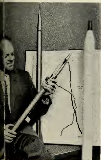
ELECTRONICS , Borg-Warner Corp. developed the Owl meteorological probe for ARDC to provide wind direction and velocity information at altitudes as high as 240,000 ft.
