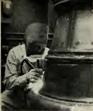
HELIARC welding the exterior of a double-walled thrust chamber for Rocketdyne's Redstone engine.
