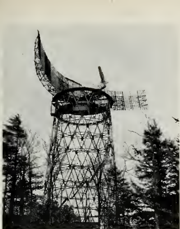
D. S. KENNEDY & Co.'s 120 ft. reflector swings continuously in azimuth at speeds up to six rpm.
