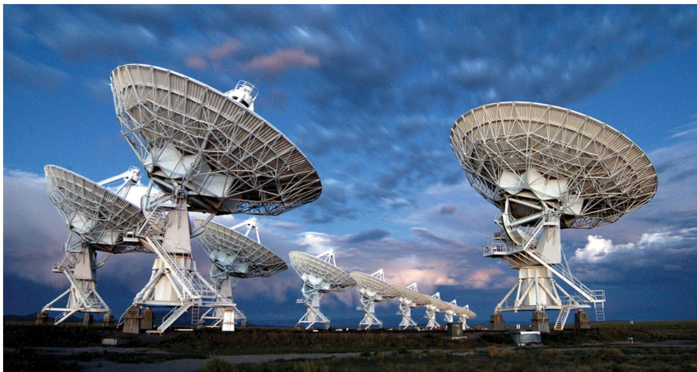
▲ **SPLITTING THE FEED** The Very Large Array is a collection of 27 radio antennas in Socorro, New Mexico. Each antenna in the array measures 25 meters (82 feet) in diameter and weighs about 230 tons. In the COSMIC SETI initiative, feed splitters will copy the data that the VLA collects, enabling special correlators to analyze astronomical data for extraterrestrial intelligence.
