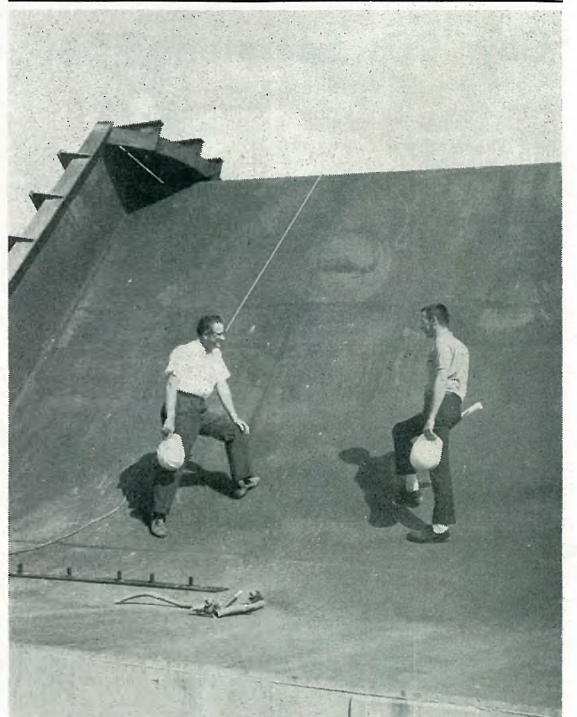
BILL QUINN, left, and Gary Richards of Facilities Operations examine Pad 34's flame deflector, which received the full fury of SA-4's searing exhaust.
