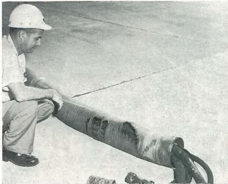
RUSSELL CLAY of Electrical Networks Group inspects post-launch damage to short cable mast.
