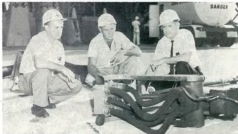
INSPECTING at close range the damage to a short cable mast on Complex 34 are, left to right, Russell Clay, John Barrow and Ike Rigell of Electrical Networks Group.
