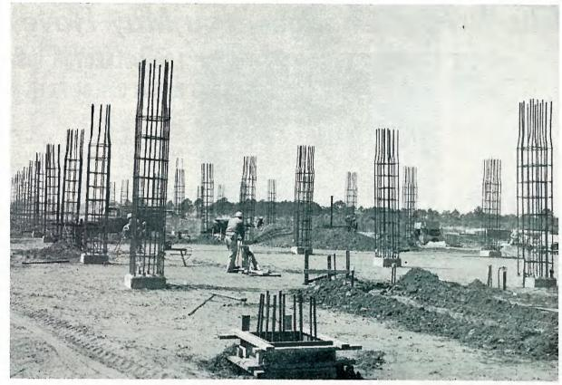
RISING UP TO PIERCE the Merritt Island skyline are these steel support ribs, which will be filled with concrete to become center posts for the Manned Spacecraft Center's Operations and Checkout Building in the MILA area.
