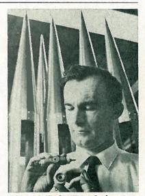
DR. LESLIE SMITH of the Geophysics Corp. of America holds solar radiation sensory instruments used on six Nike-Apache sounding rockets fired into the ionosphere from Ft. Churchill, Canada, during the solar eclipse.
