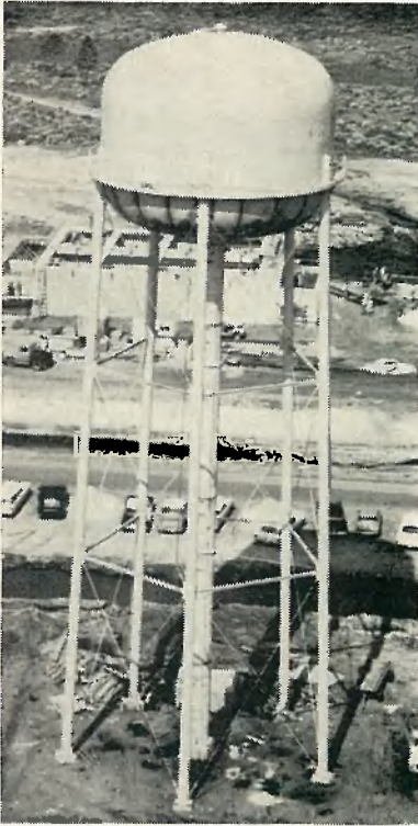
TOWERING high over the Merritt Island Launch Area landscape is this 250,000-gallon water tank, which along with a ground-level million gallon tank will service MILA's water needs.
