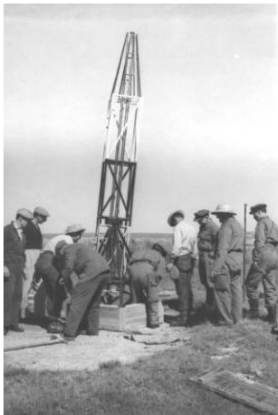
Figure 3-4: Argentine Air Force personnel installing the Alfa-Centauro launch tower. Author's Archives.
