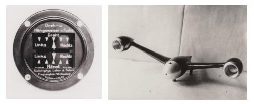
Figure 1–7: Flight altitude control instrument 1936/1937 on behalf of the Austrian aircraft manufacturer Wr. Neustadt.
