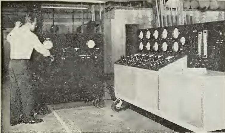
A substantial number of these mobile pneumatic and electrical test stands (right) have been produced by Lear Aircraft Engineering Div., Santa Monica for North American Aviation's Rocketdyne Division to check out rocket engines without firing. Complexity and high-performance requirements of their operation led to design of another auxiliary test stand (left) to check them out.
