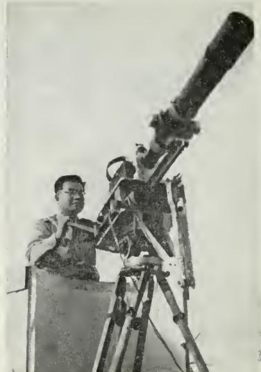
Photo-theodolite tracking rockets.
