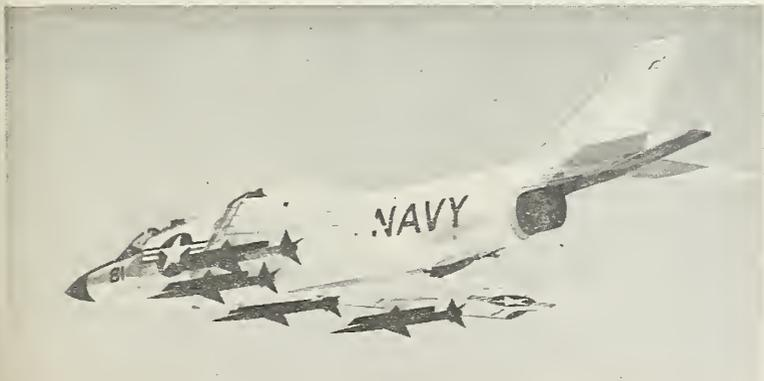
McDonnell Aircraft's F3H-2M, missile-carrying version of its Demon all-weather fighter, has passed all Navy trial and evaluation programs required for fleet release and joined operating squadrons. New Demon carries four Sperry Sparrow air-to-air missiles plus rapid-firing, high-velocity 20mm cannon. Powerplant is Allison J71 jet. Both F3H-2M and F3H-2N all-weather fighters are slated for production through March 1958.
