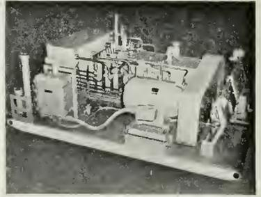
New "central compression system" developed by Cardox Corp. for testing aircraft and missile pneumatic systems delivers 54 acfm of air with  $-70^{\circ}\text{F}$  or lower dewpoint at any needed pressure from 3,000 to 12,000 psi.
