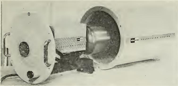
A new ruggedized camera developed by Kay Lab for rocket and jet engine test facilities and rocket launching sites has been designed for high-noise applications.
