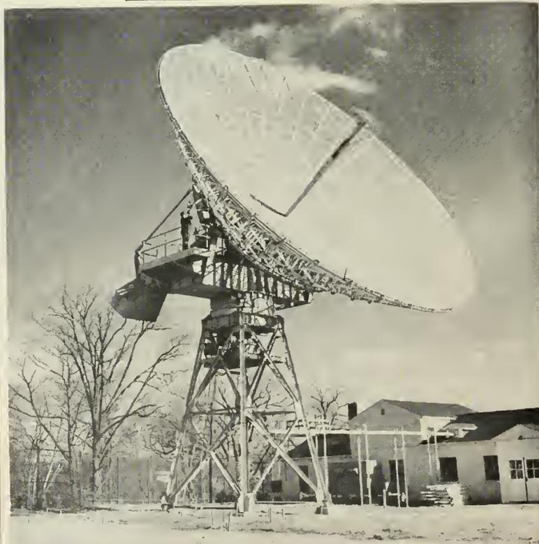
This Army Signal Corps DIANA moon radar has been used recently to bounce signals off the moon in efforts to develop a technique for the testing of VANGUARD and other satellite tracking stations. The unit may be used in calibration of MARK II stations.
