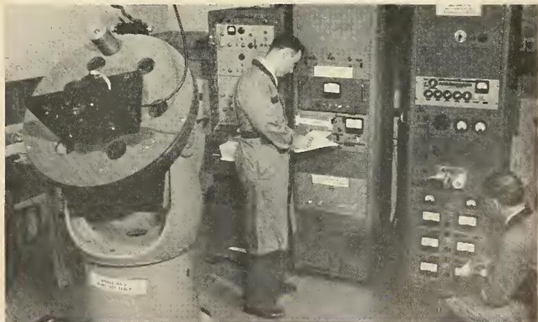
Engineers examine air-bearing gyro drift data that has been recorded by drift-rate measurement apparatus. Equipment will measure angular drift rates of one revolution in 40 years.
