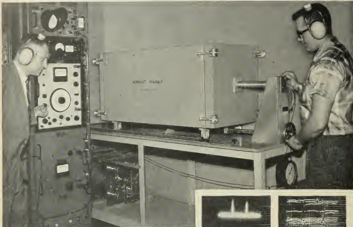
L to R: Dr. Fricke, Engineer-in-charge Acoustics Laboratory, and Mr. Kuzara Acoustics Engineer, evaluating a component in a high intensity acoustic environment. RIGHT: Malfunction of a relay at high-intensity sound as disclosed in a sound chamber.
