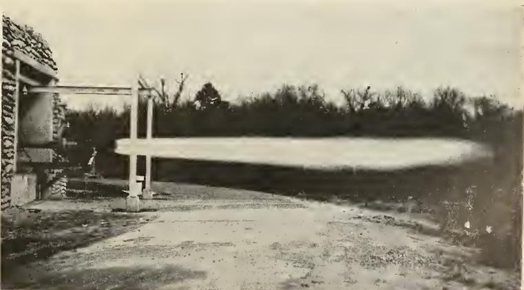
The long flame produced during a static firing of the NIKE-HERCULES sustainer motor is indication of a high thrust level. Cooling is so effective motor units may be re-used.
