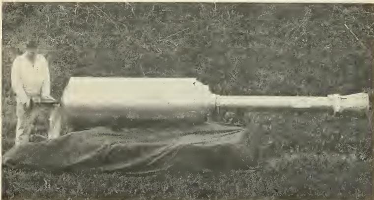
The NIKE-HERCULES sustainer motor is an uncooled and long burning unit. Success of the motor is due to advances in insulation techniques by Thiokol and Haveg Industries.
