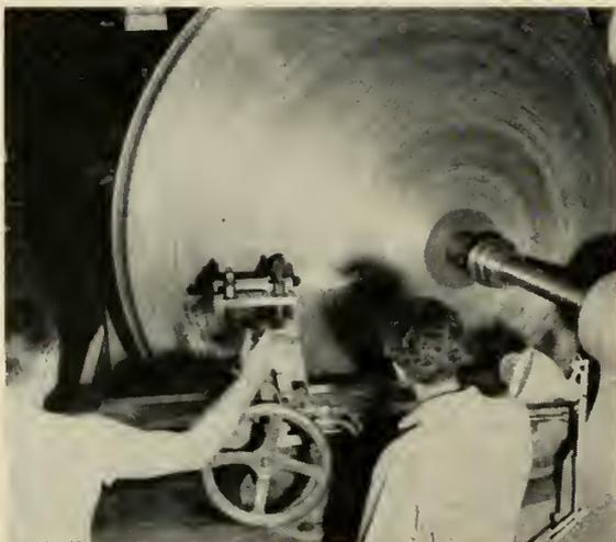
Cold spinning  $\frac{5}{8}$ " aluminum alloy to an 8' finished part for ICBM pressure bulkhead. Used here is Model Plb 1200 hydraulic spinning and planishing lathe. German manufacturers are Leifeld & Co.
