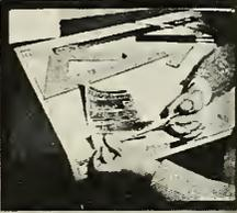
2 PLACE the tri-ocetate in position on the tracing.
