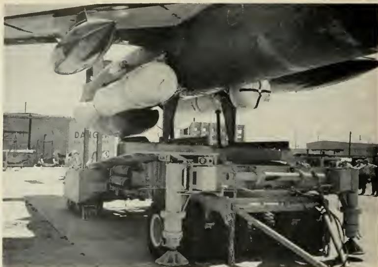
SNARK zero-length launcher which could be used on carrier.
