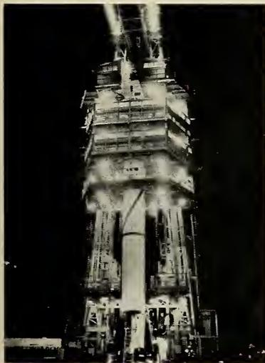
January 31st — With countdown for launching under way and proper weather conditions assured, last minute checkouts induced unwarranted tensions. Fuel spillage caused several minutes delay when leakage was suspected. At countdown "zero" missile pressurization was started. Ignition started at X plus 14 seconds. The rocket took off at 15.75 seconds after "zero."
