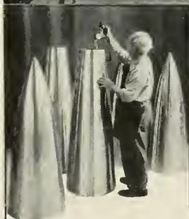
Nose and aft sections, Phoenix fabricated
