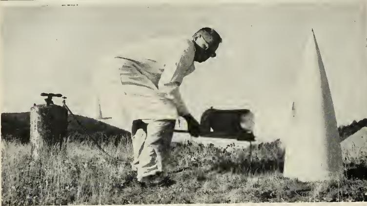
**BLOWTORCH demonstration of the heat resistance of a glass-ceramic radome.**
