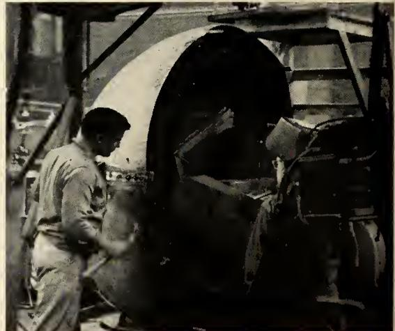
**SEGMENTS** of the hemispherical head are being fitted together on a welding positioner. Tanks such as these will accompany *Thor* squadrons overseas (to Britain) this fall.
