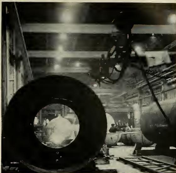
**STAINLESS STEEL** inner shell sub-assemblies for huge tanks. Automatic welding head in the upper foreground is an example of the kind of fabrication required.
