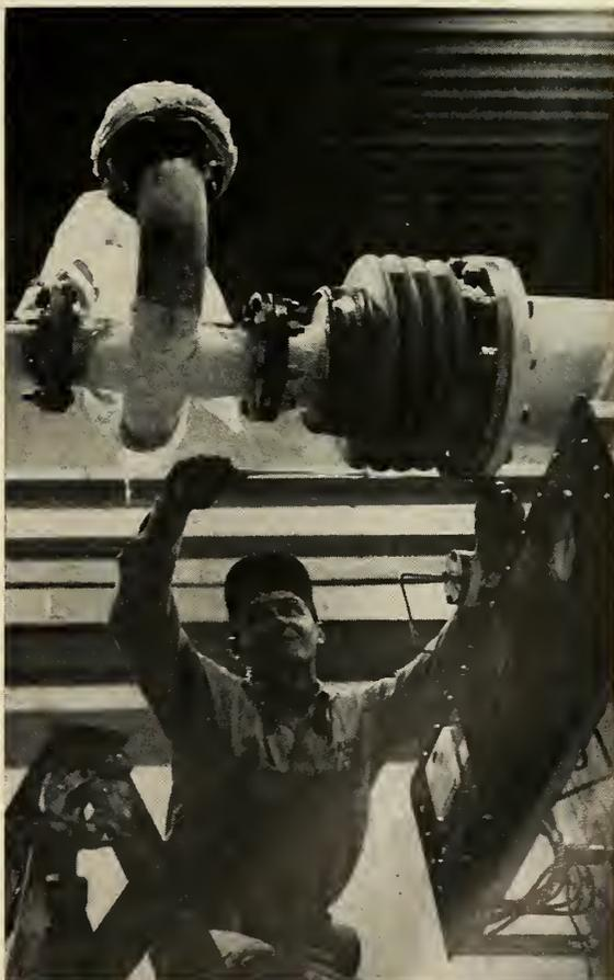
**VENT LINE** expansion bellows must be carefully inspected during liquid nitrogen run-down test. Note the ice that has formed on the equipment. Tank is ready for shipment.
