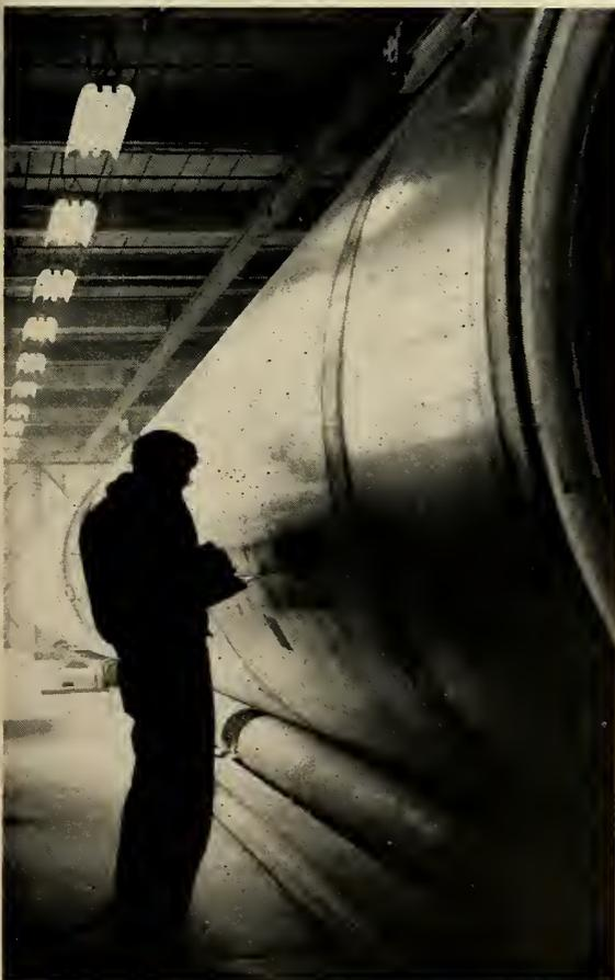
**THERE CAN BE NO LEAKS** in the evacuated area between the two shells. Here, an inspector checks the condition of welds in the outer shell of aluminum plate.
