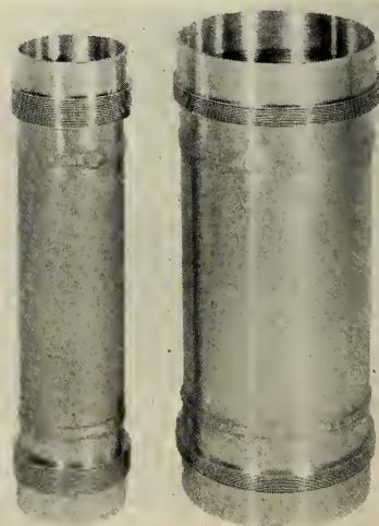
seal machined on each end, permitting high pressures. The joint also permits extremely high and low temperatures—the latter to  $-320^{\circ}\text{F}$ .
