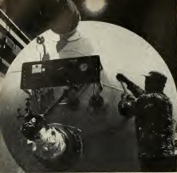
**HERE ARE THE WORLD'S LARGEST** airborne storage vessels. The business end of *Thor's* 13,500 gallon capacity liquid oxygen loading tank shows the size of the fabrication job. Cambridge Corp. builds tanks for Douglas Aircraft.
