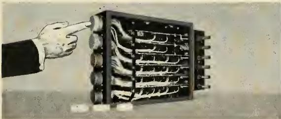
**Emergency Fire Control**—Used in the Flight Engineer's console of the Douglas Globemaster, plunger actuation allows instant emergency operation of any or several of the following: prop feathering, closing cowl and oil cooler doors, stop fuel and electrical service, fire extinguishing system actuation. Unit illustrated handles six distinct areas with instant cancellation of command feature for error correction.
