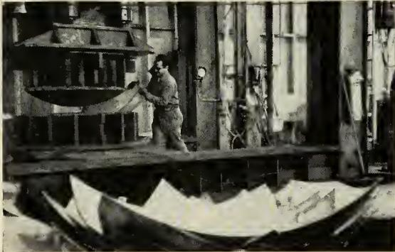
**SEGMENTS** of tank's hemispherical heads are formed by a 500-ton hydraulic press. These LOX tanks are giant double-shell dewars with a high vacuum between the shells.
