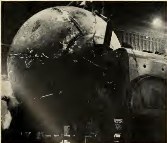
**SPECIAL JIGS AND FIXTURES**, such as this welding positioner, are needed in assembling stainless steel inner and aluminum outer shells.
