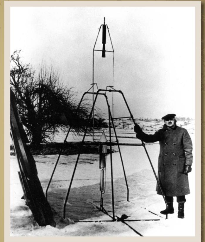
“I imagined how wonderful it would be to make some device which had even the possibility of ascending to Mars,” thought 17-year-old Robert Goddard in 1899. In the Massachusetts snow on March 16, 1926, he took the first step by developing and launching the world's first liquid propellant rocket. Photo credit: NASA
