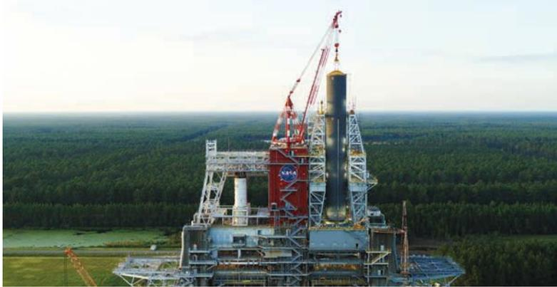
▲ **The Space Launch System's** core stage pathfinder is positioned in the B-2 Test Stand at NASA's Stennis Space Center in Mississippi. Crews practice handling skills with a pathfinder before working with the real core stage.
