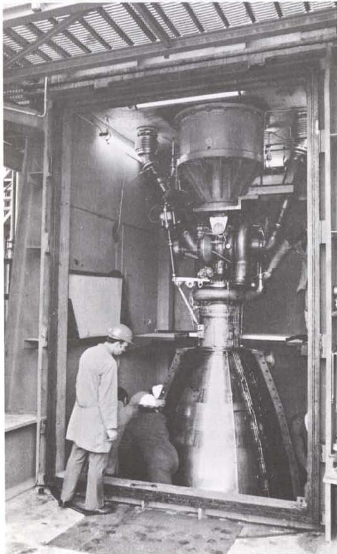
Figure 3 – Ariane's second-stage engine being readied for test (test stand P4.2).
