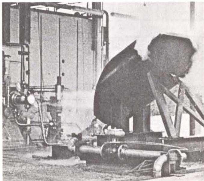
Figure 9 - Thrust-unit test stand.
