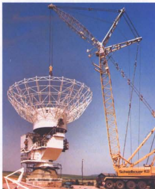
Figure 4. Construction of the 15m-diameter Meteosat antenna (for data acquisition, telecommand and tracking), in the Odenwald, W.Germany
