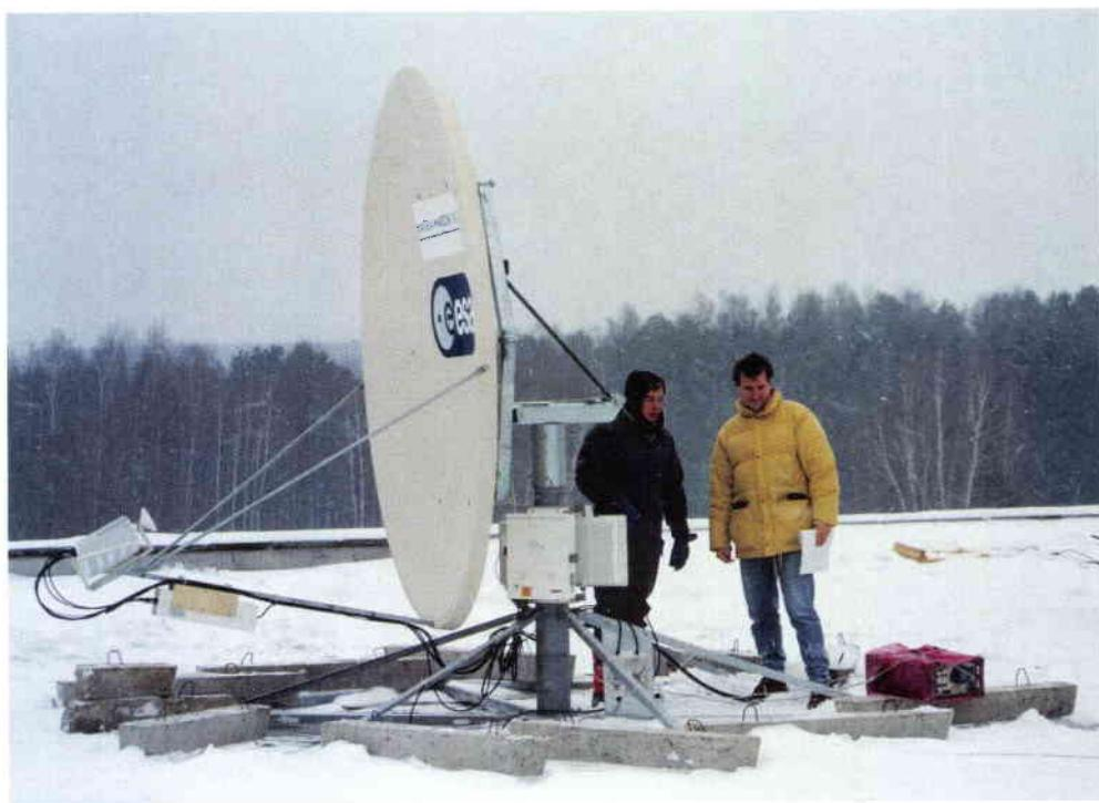
**Figure 2. A DICE Earth station being installed near Moscow**
