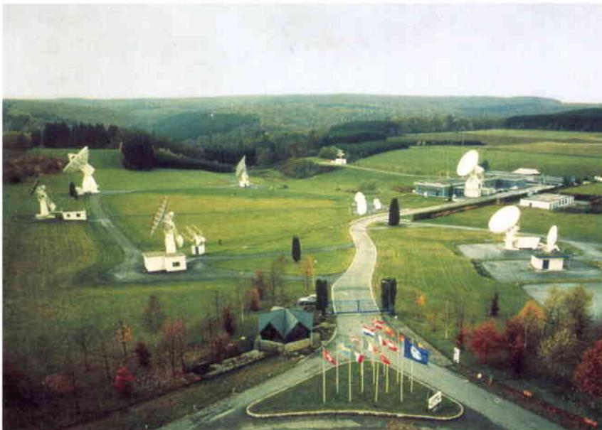
**Figure 5. ESA's Redu (B) ground-station complex has been equipped with a new 15 m antenna (on extreme left of photo) and associated equipment to support Cluster operations in S-band**
