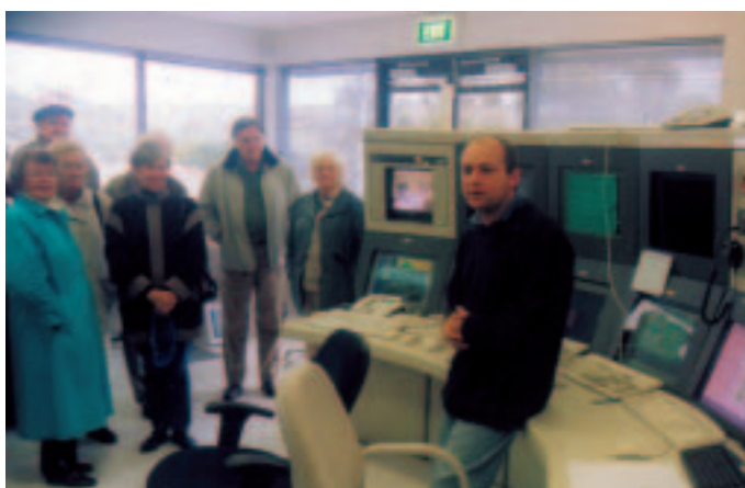
Brett Schipp explains the control room
