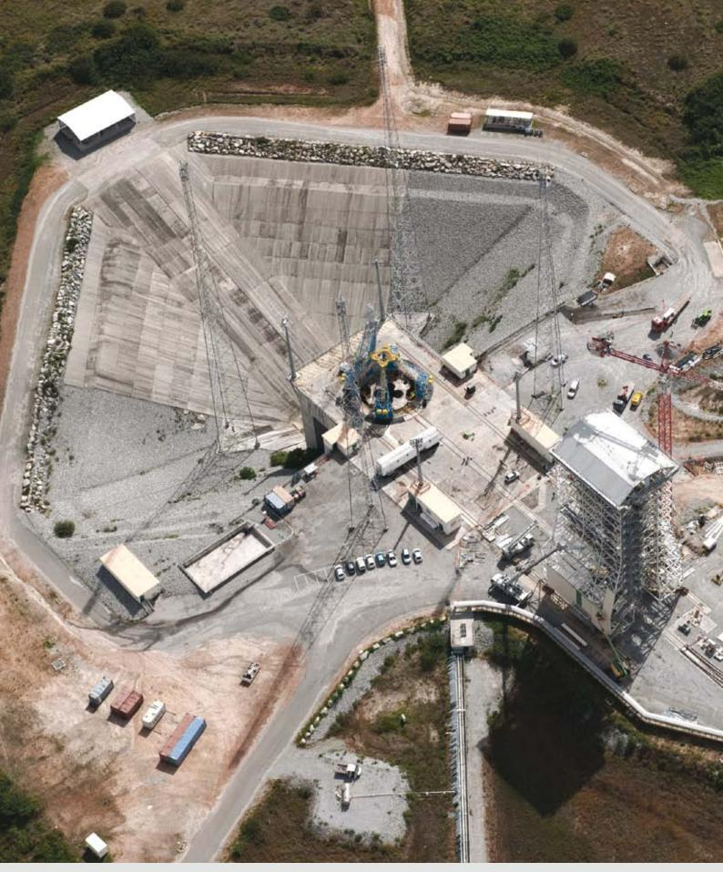
The new Soyuz launch facility at the Centre Spatial Guyana (CSG), Europe's Spaceport in French Guiana, with a view of the Soyuz launch platform from the flame pit. This five-level reinforced concrete structure houses mission equipment. The top two levels have 15 m-wide openings for the launch table and the erected Soyuz vehicle. Its upper area accommodates the pad infrastructure, including the service tower, the fuelling booms and the erector (ESA/CNES/Arianespace/Optique Video CSG)
