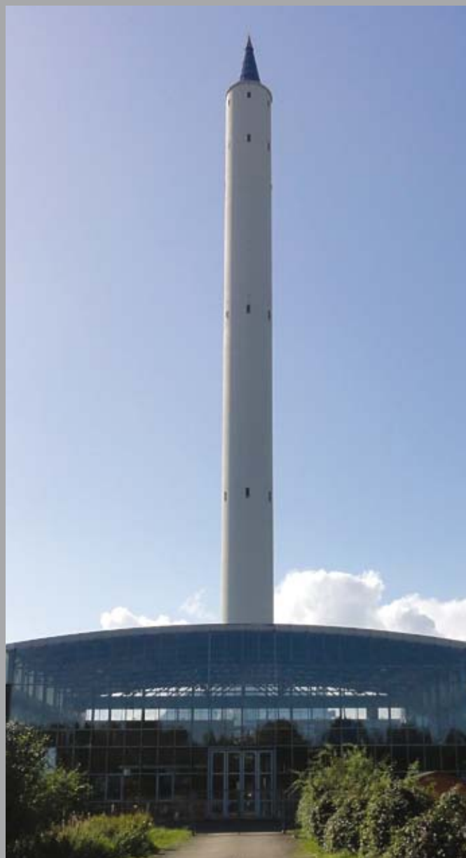
The 146 m ZARM drop tower, at the University of Bremen, is one of the tallest and best-known drop tower facilities in Europe and the home of ESA's 'Drop Your Thesis' campaigns (J. Howaldt)
