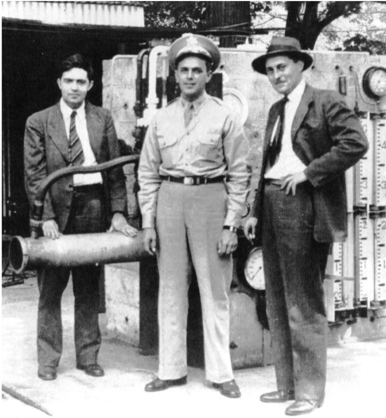
Figure 5-12: Wyld, at left, with an unidentified officer, and Lovell Lawrence, Jr., at right, with a vastly improved and more powerful 3,000 lb (1,360 kg) single-chambered RMI regeneratively-cooled motor, ca. 1944 or 1945. Note also, the greatly improved stationary test stand, although it still utilized elements, like the vertically-mounted glass propellant volume level gauges, at right, adopted from the original portable ARS Test Stand No. 2. Original ARS Test Stand No. 2 dials may have also been “borrowed.” The Navy was always RMI’s biggest war-time customer and these large motors were meant as critically-needed Jet-Assisted-Take-Off (JATO) units for heavily-loaded airplanes for operating from Pacific islands in the Pacific Theater. Photo, originally from the Frederick I. Ordway collection. Smithsonian Photo 89-1847.
