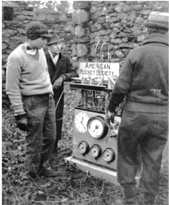
Figure 5-6: James H. Wyld, left, besides ARS Test Stand No. 2, and other ARS members Joe Battaglia, middle, and John Shesta (back turned), at right, in preparation for the second series of tests with Stand No. 2, within an abandoned house foundation at New Rochelle, New York, on 10 Dec. 1938. This series was to include Wyld's motor—the first time it was ever tested—although the motor is not shown on the stand in this picture. Photo donated to the NASM by Wyld's sister, Mrs. Anne W. Blizzard, Washington, D.C. Smithsonian Photo 92-17120.
