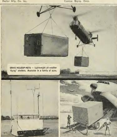
OBSERVATION-DOMEO SHELTER with 4-wheel dolly for air traffic control and other operation.
