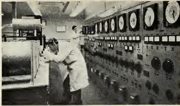
HEAT TREATING furnaces at Nuclear Metals, Inc., where "exotic" metals are investigated for high temperature resistivity.
