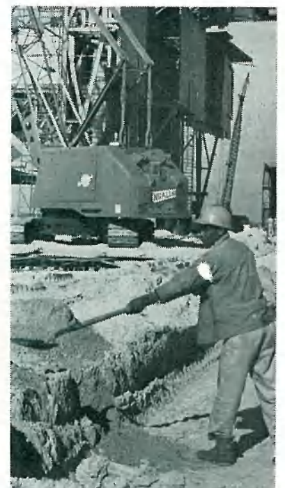
A LONE shoveler digs path where rails will be laid.
