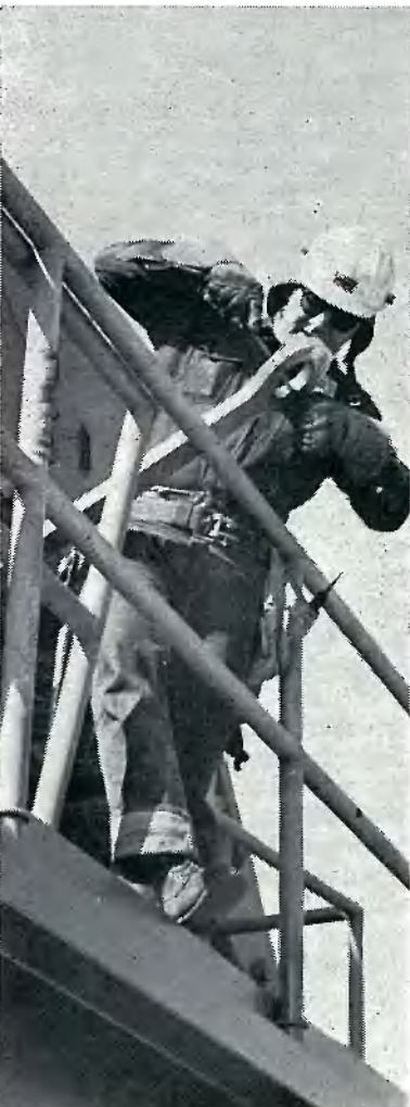
ON TOP of 37's tower a worker files steel eyelet.
