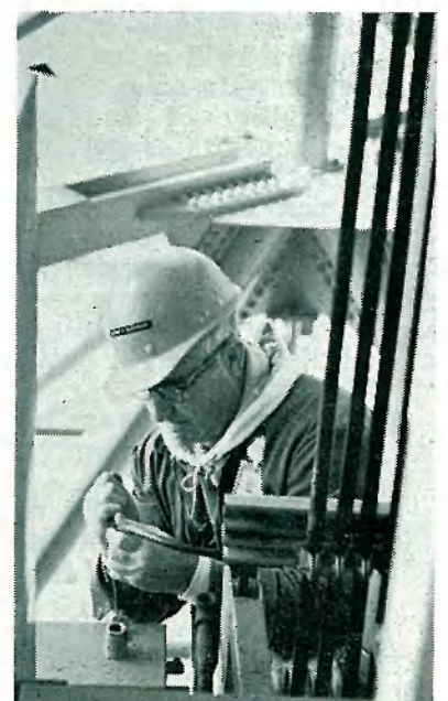
HIGH in the tower an electrician "skins" wiring.
