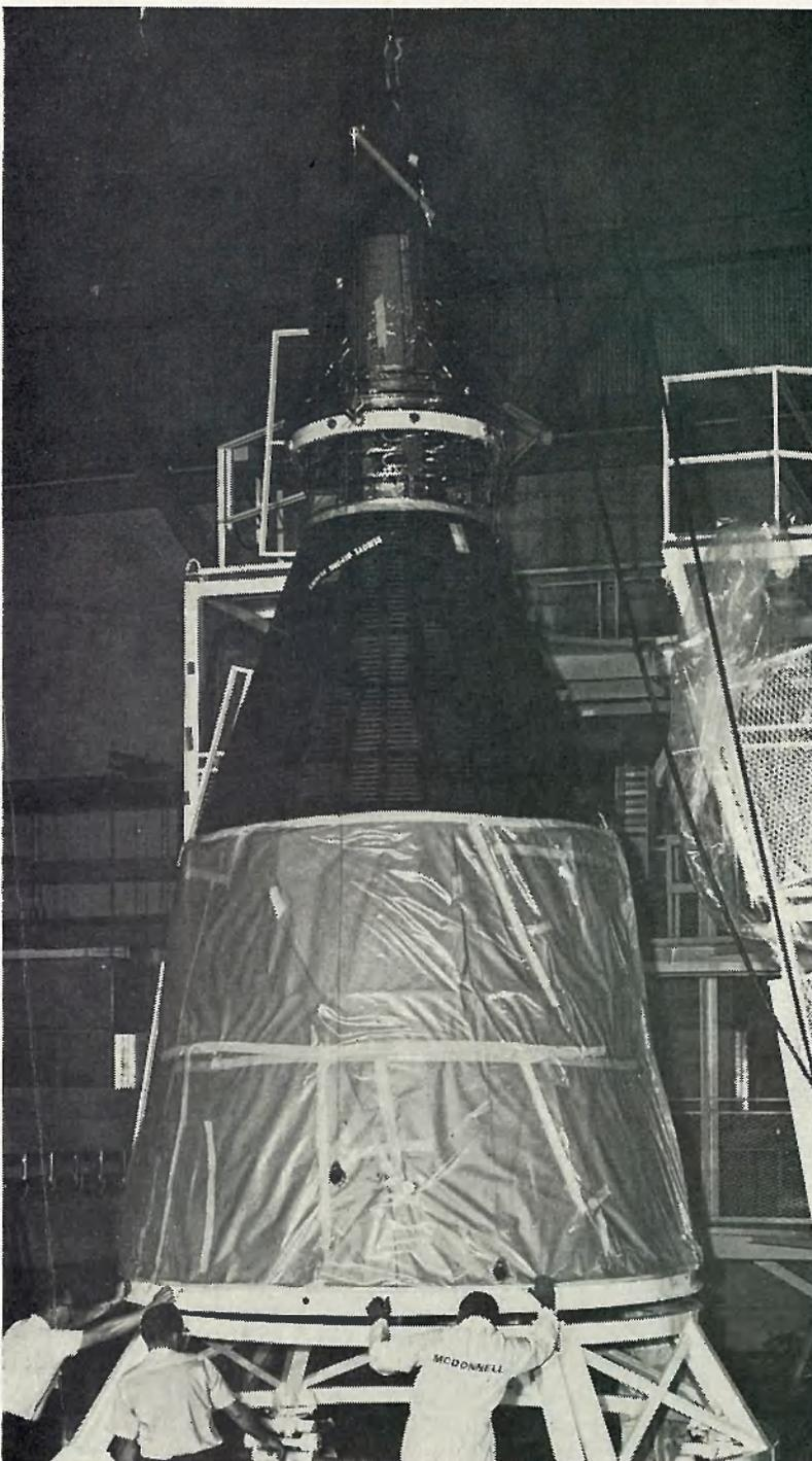
**TECHNICIANS POSITION** Gemini spacecraft into its stand in Hangar AF following its Cape arrival Friday. The capsule will undergo thorough checkouts prior to flight.
