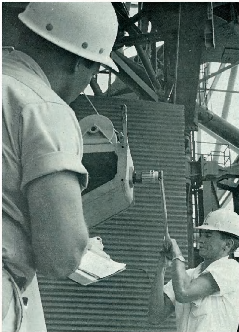
WHILE George Hughes of KSC supervises, Chrysler mechanic Dave Wiggins checks a torque on the holddown arms.
