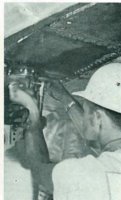
A PAD mechanic makes modification to pad's water quench brackets.
